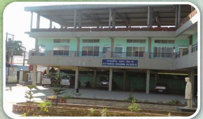
Extended Building Block A during Construction
